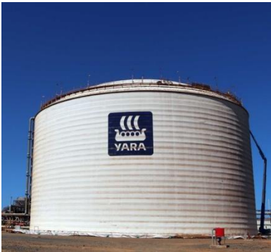
Ammonia storage tank 150 GWh storage capacity
