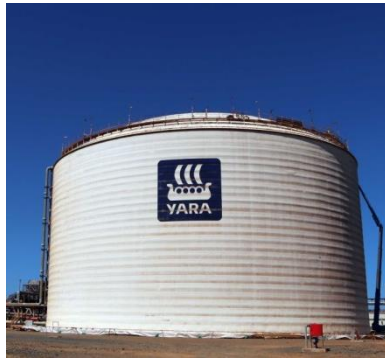
Ammonia storage tank 150 GWh storage capacity
